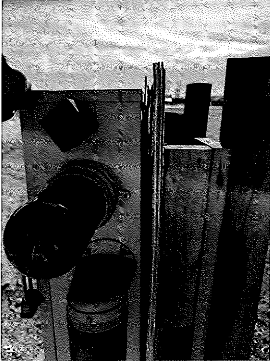
Figures 4. Panel not secured to plywood.
