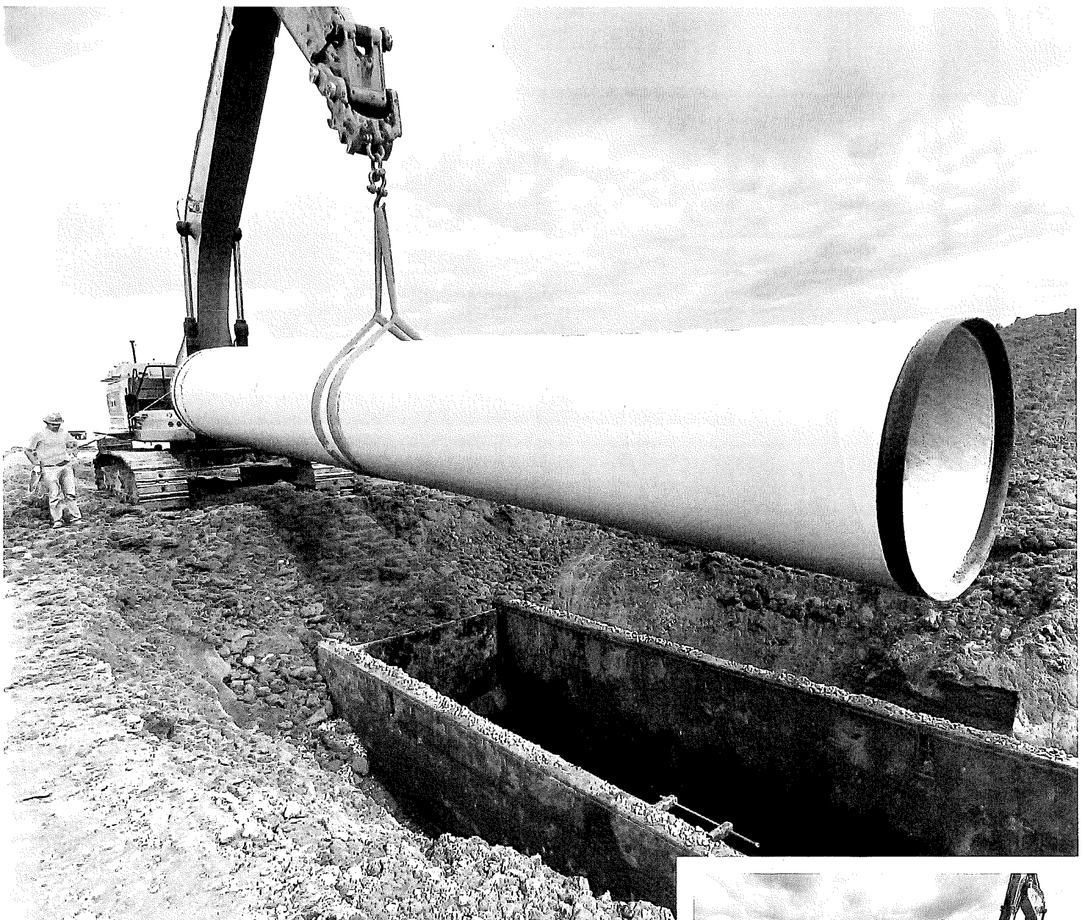
The spiral-welded steel, concrete-lined and epoxy-coated pipeline is 6 feet in diameter.
