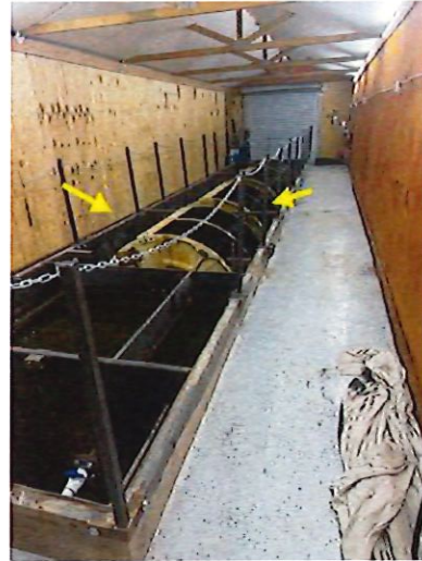
Consider adding guardrails for safety.
