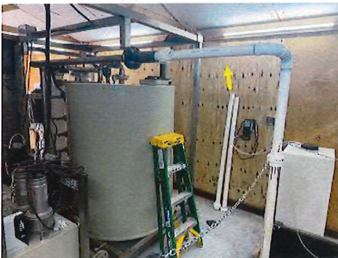
Pipe over walkway.
