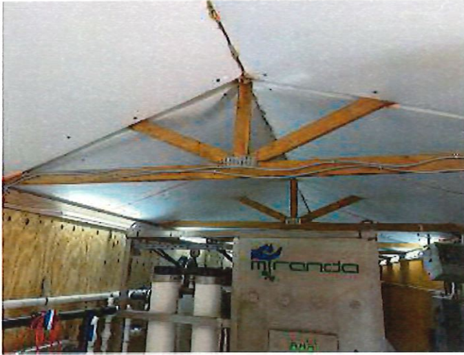
Truss type rafters.
