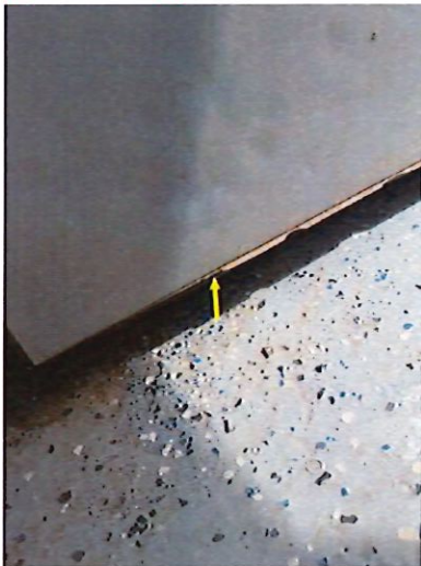
Weatherstrip damaged.
