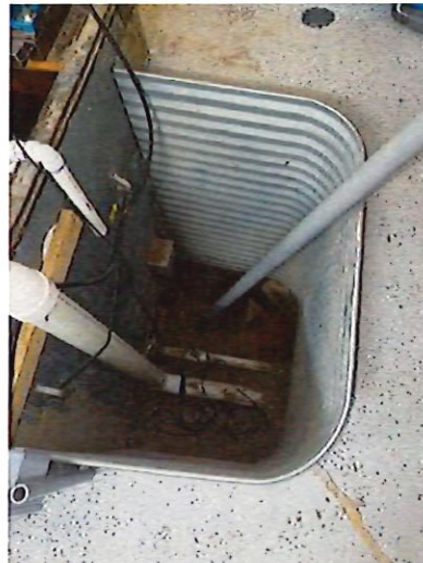
Open well at back of building.
