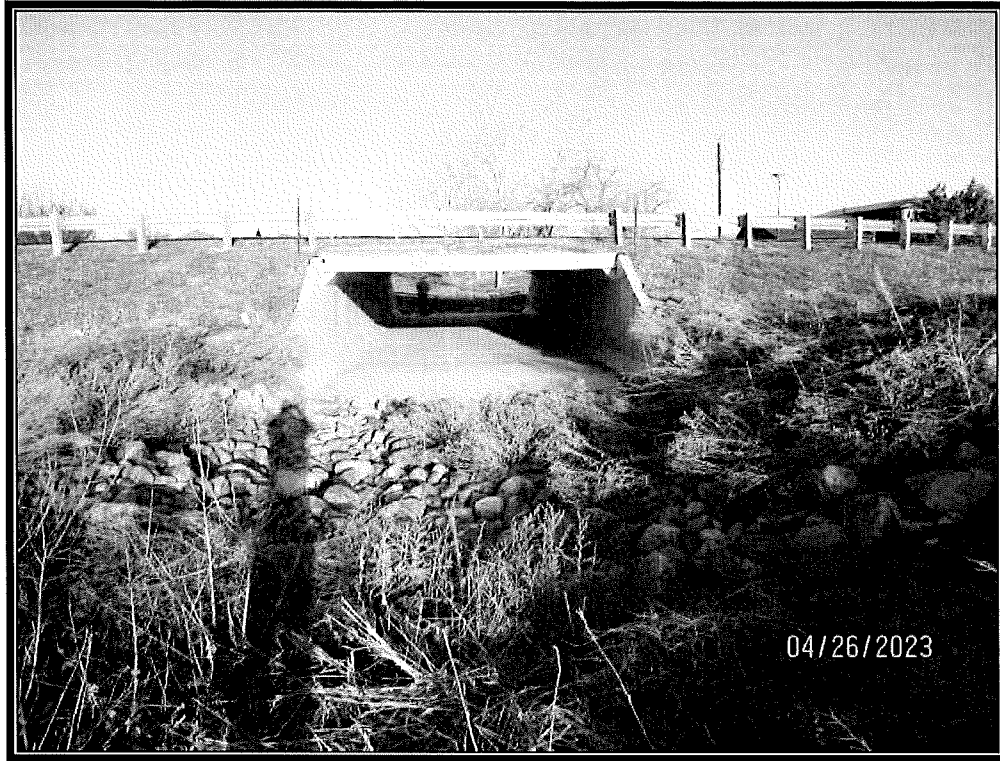
Downstream Looking West
