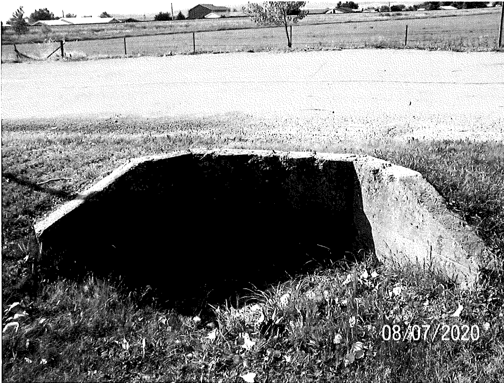
INLET END OF 2'X4' BOX CULVERT
