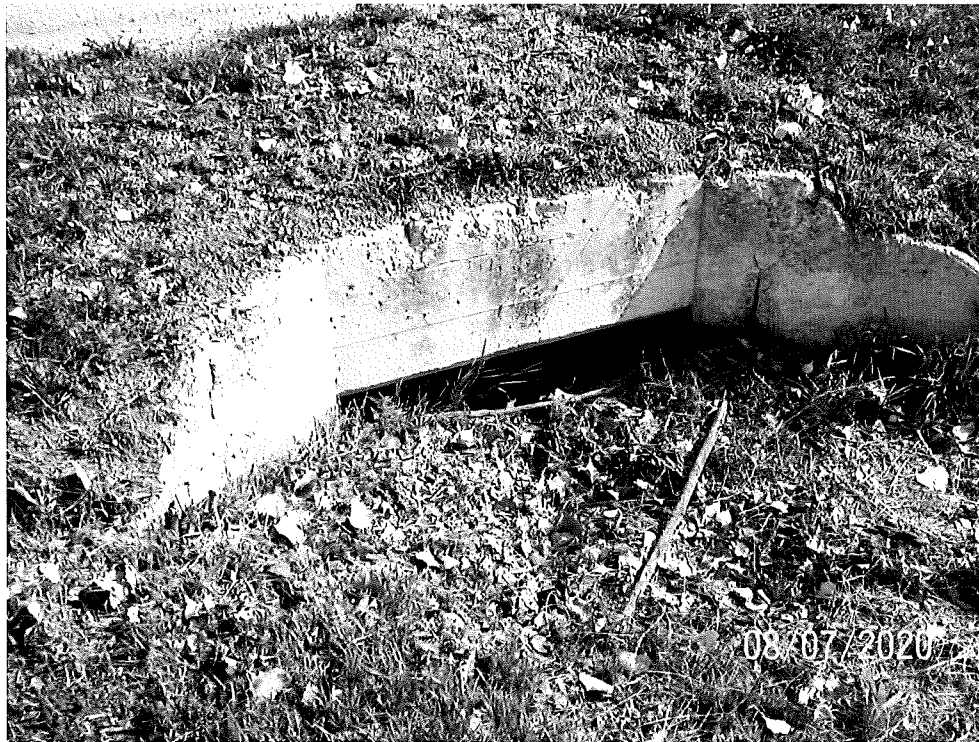
OUTLET END OF BOX CULVERT
