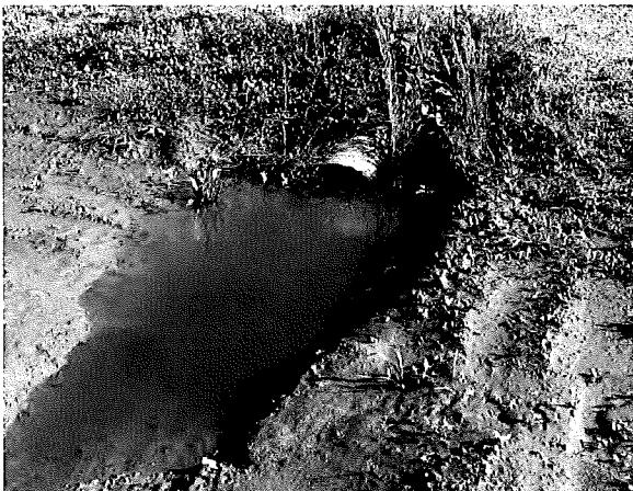
Photo 2: Marie Street 18" CMP Outlet partially submerged.
