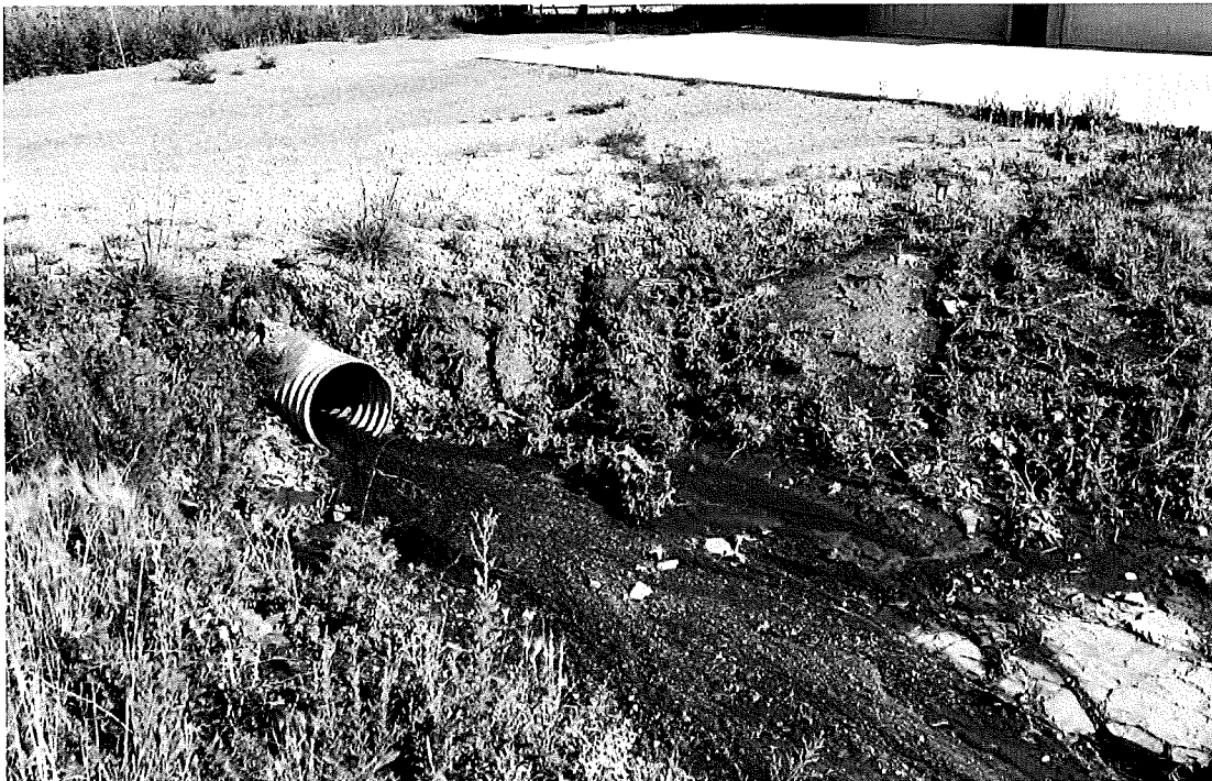
Photo 6: Culvert outlet showing a high level of sedimentation in ditch with sparse vegetation, view NW
